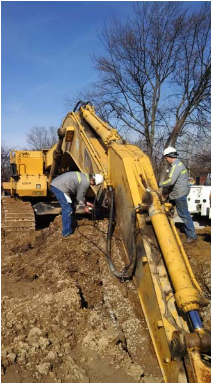
Louie Rouse and Glen Petty assembling the 385 CAT excavator on US 31.
