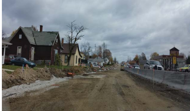
US 40 in Brazil ready for pavement and curb.
