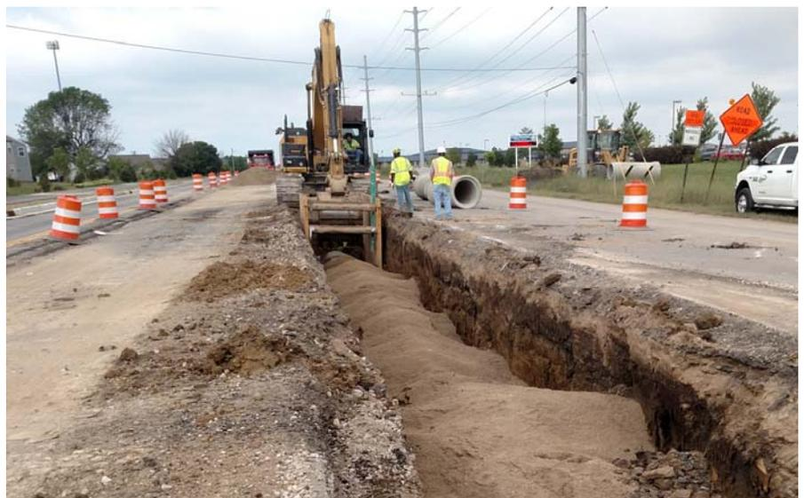
Operator Zach Morris and laborer Mike Ellington from Matt Burton's crew installing 30" RCP in the median at Worthsville Road with INDOT inspector looking on. In the background on the loader is operator Randall Shipman.
