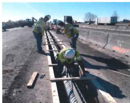
Matt Burton's crew installing slotted drain on the Worthsville Road project.
